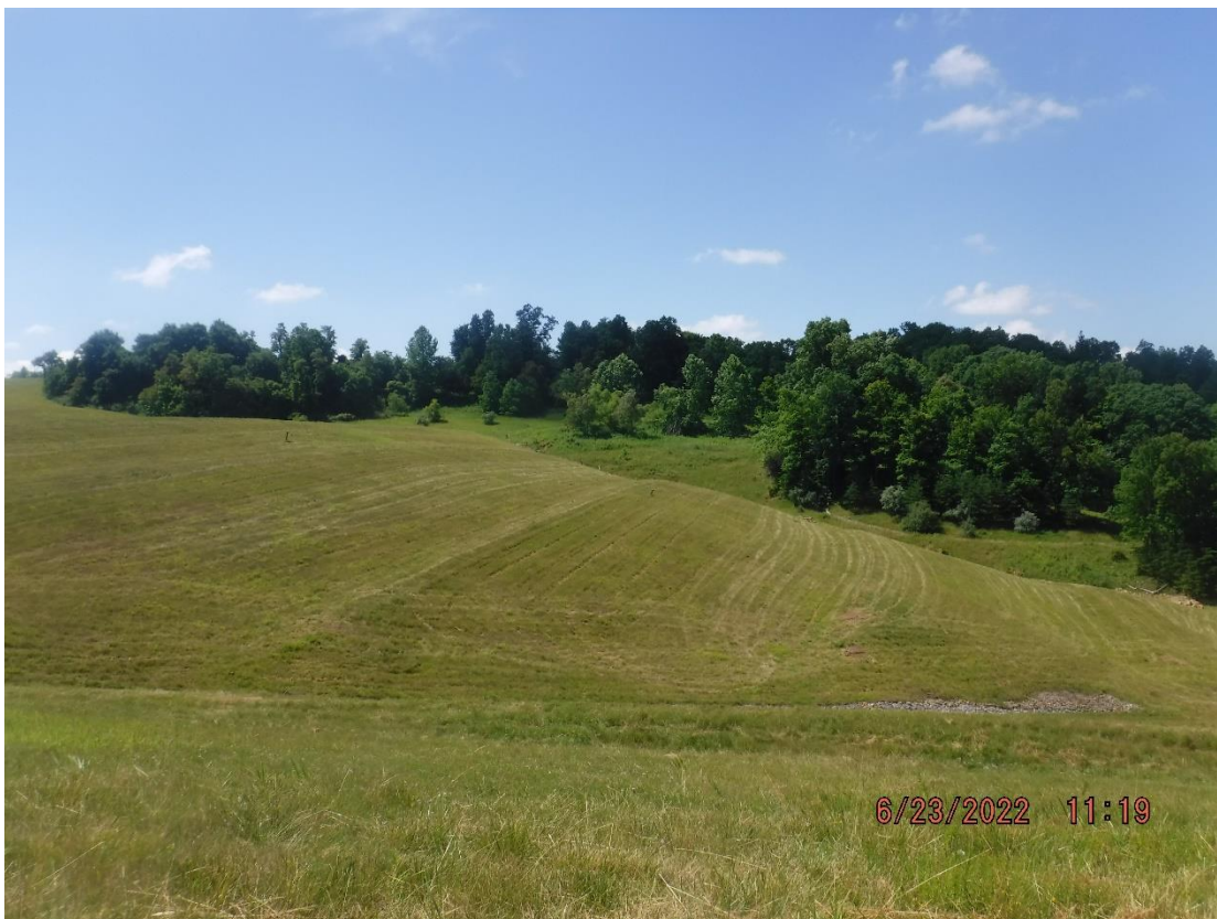
Landfill overview – 6/23/2022 11:19 am
