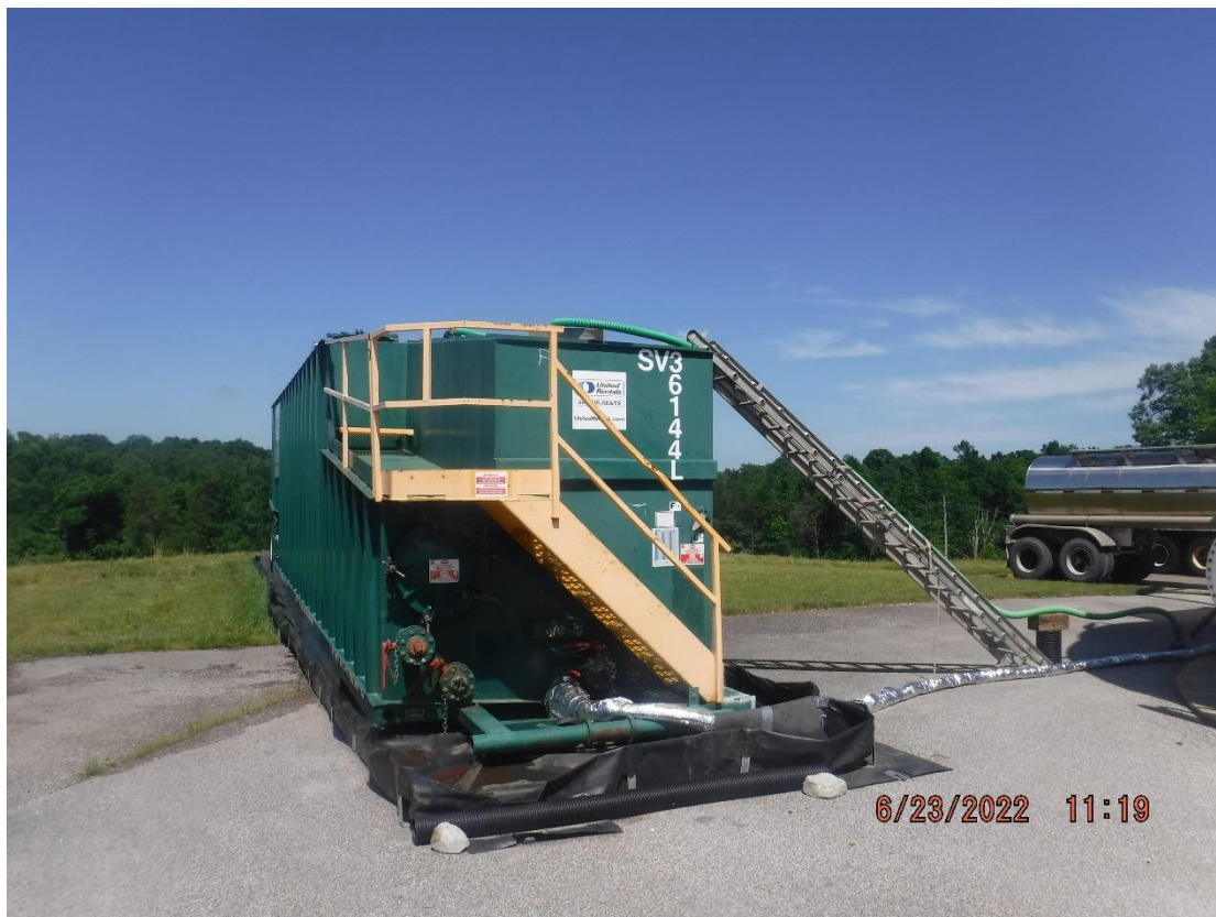
Leachate is temporarily being stored in a frack tank – 6/23/2022 11:19 am
